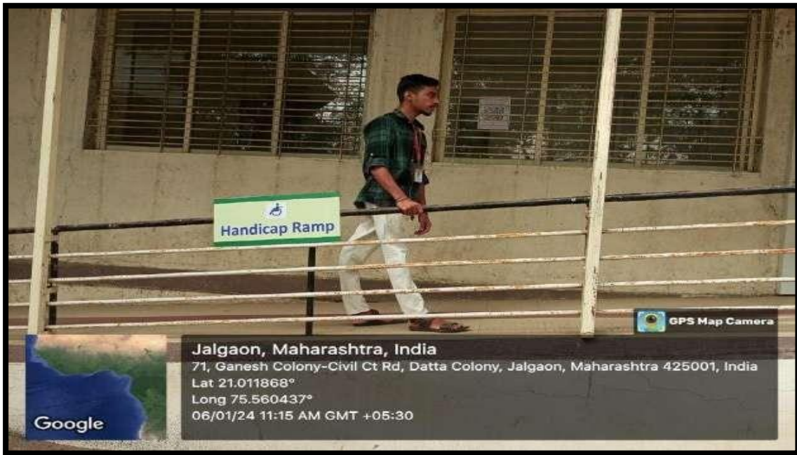
Ramps made available to approach Principal office and Administrative office
