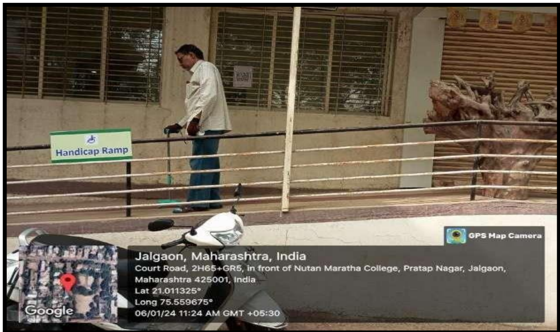
Ramps made available to Administrative office
