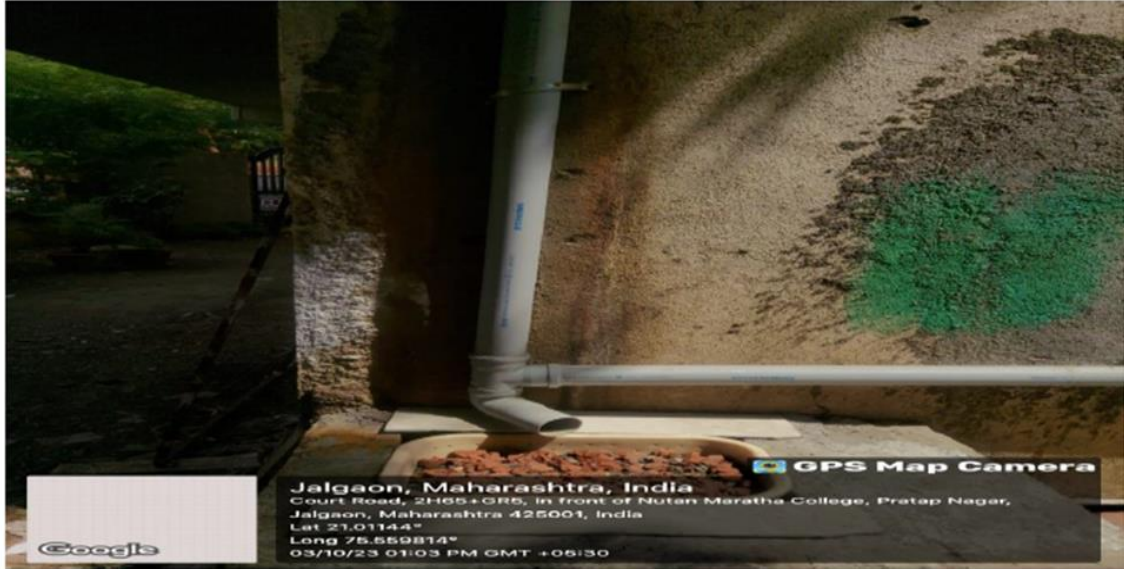
Chemical Collected in Drainage Tank
