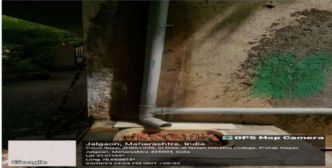
Chemical Collected in Drainage Tank
