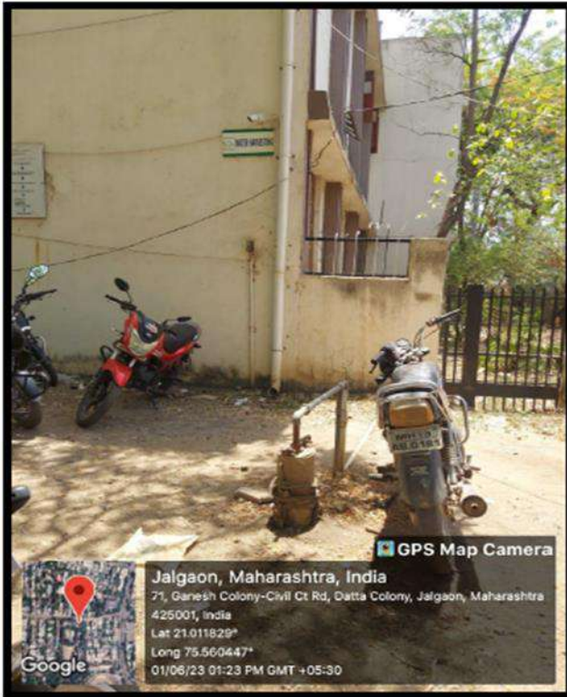
campus building roof area water Collect then we Borewell Recharge System
