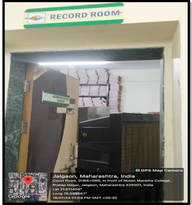
LED Tube lights in and Record room
