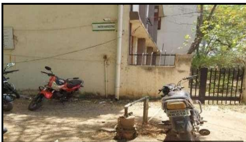
Rain Water Harvesting Area
