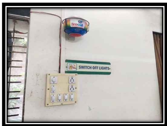
Fire extinguisher Ball and cylinder
